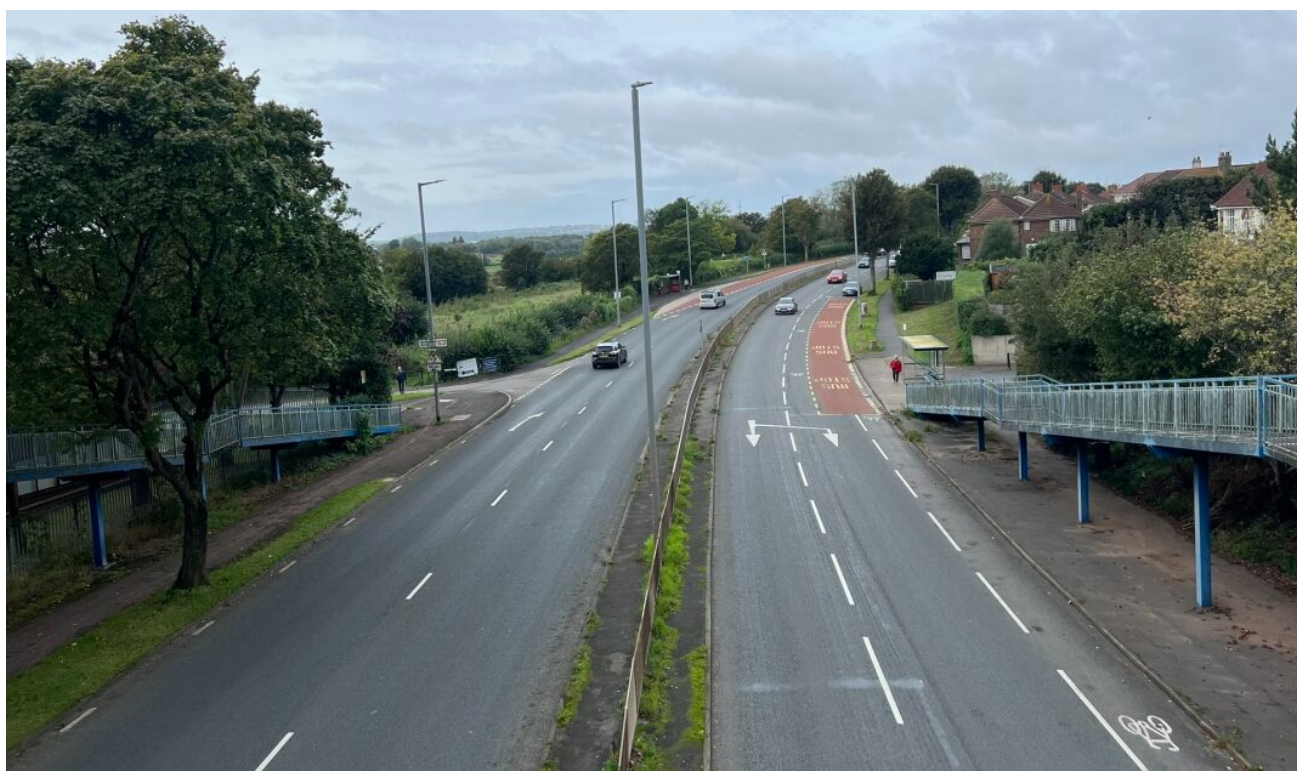
Figure 2-16 - Photo of carriageway cross-section near Shirehampton Station
