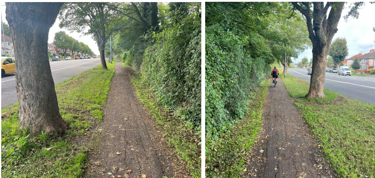
Figure 2-8 Photos of narrow footway/cycleway between Shirehampton and Portway Park & Ride
