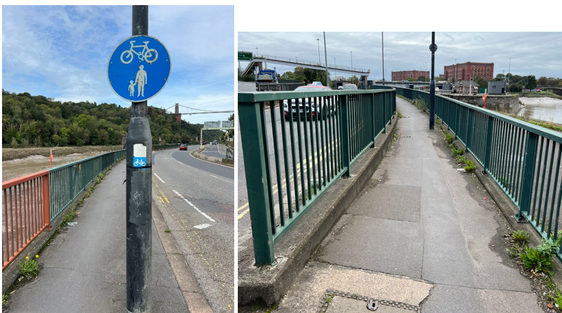
Figure 2-9 Narrow, obstructed shared footway/cycleway on Hotwell Road
